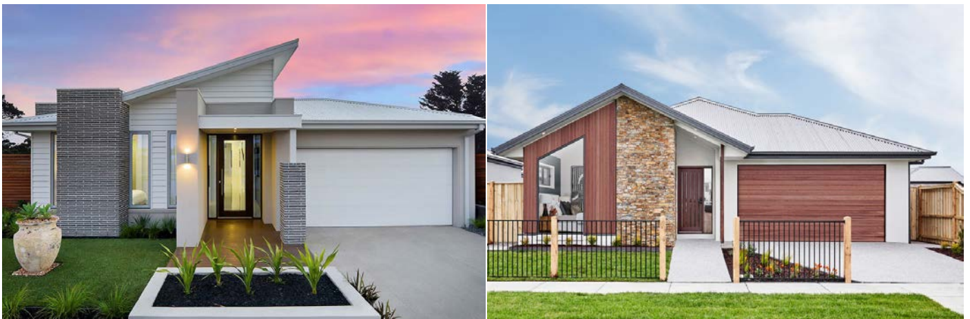
Above: The front façade must include at least two different wall materials
